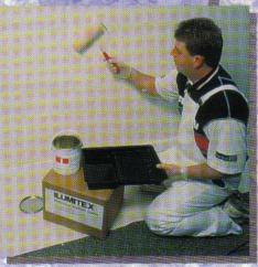
When surface is dry rub down or use a stiff brush and apply the lacquer with a short pile roller or brush.
