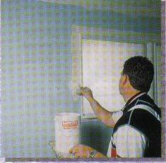
The Base coat (which acts as an adhesive to receive the flakes) is applied as a thick even coating by brush/roller.
