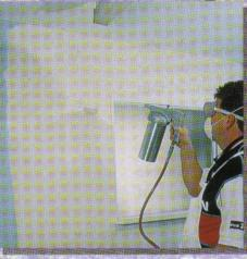
Holding the gun 12 - 18" from the surface, spray the flakes using slow horizontal and vertical passes until the required surface is fully covered.\*
